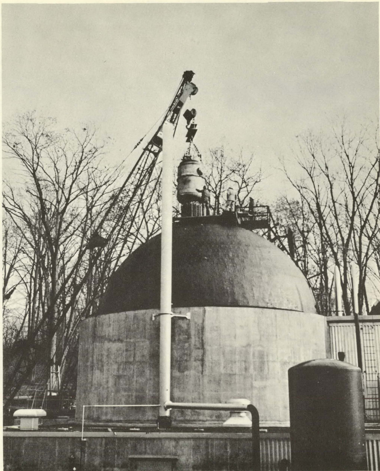
FIG. II - 2 REACTOR VESSEL BEING LOWERED INTO VAPOR CONTAINER
